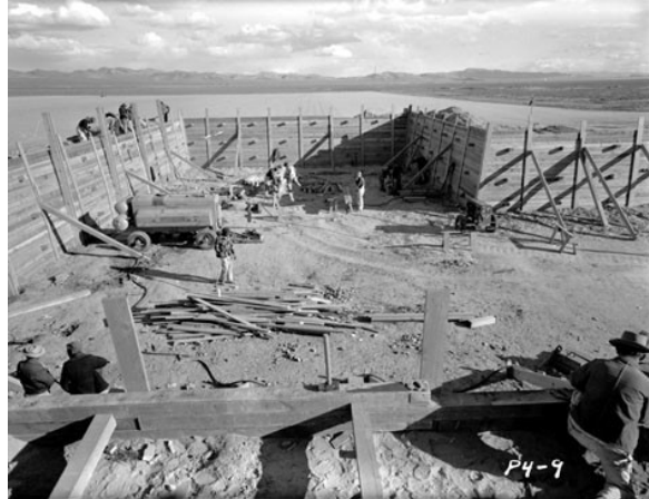
Russian revetment under construction
